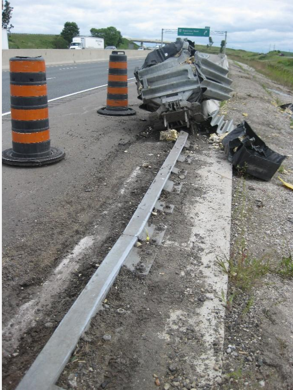
View of fully-compressed end-treatment to a New Jersey barrier as a result of the bus impact.
