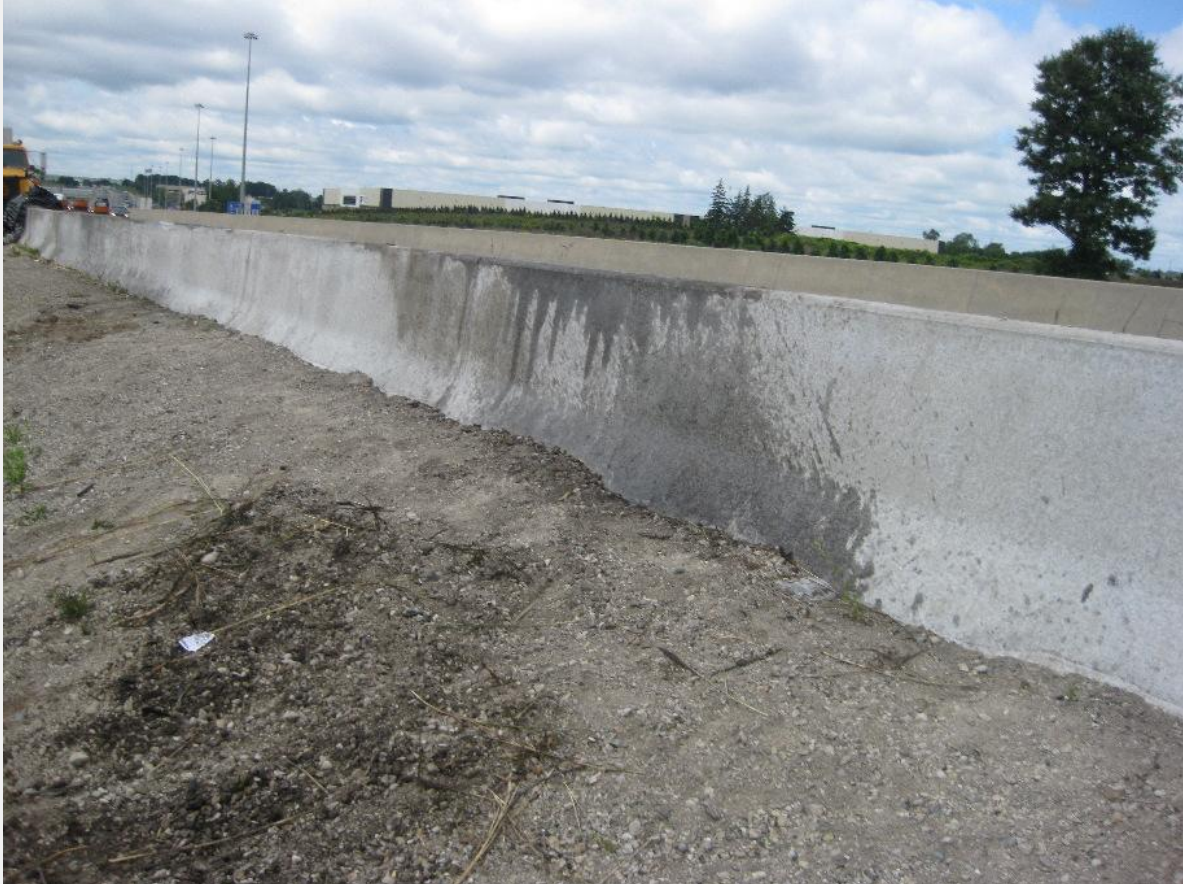
View of oil stain the New Jersey barrier indicating that the bus slid over top of it before rolling over.
