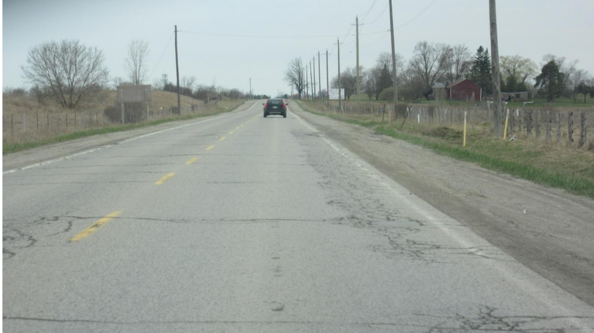
Figure 4: View, looking westward along Fanshawe Park Road in the fall of 2019 showing the poor road surface just west of Clarke Road.
