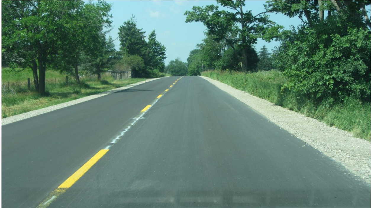
Figure 6: View looking west along Sunningdale Road west of Clarke Road just after its re-surfacing on July 11, 2019.
