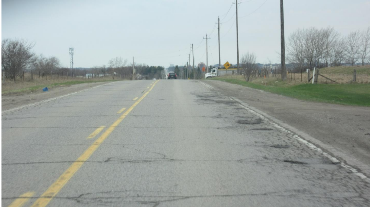
Figure 5: View, looking west along Fanshawe Park Road in the fall of 2019 showing the poor surface just west of Clarke Road.
